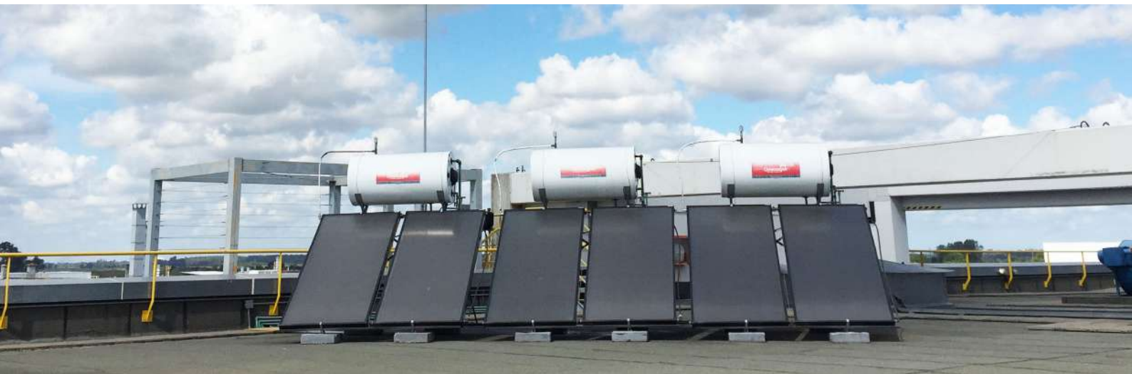
Thermo-panels in Zarate Plant buildings
